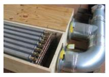
**Figure 211:** Phase Change Material based air tempering system. Detail of the closed ducts system. Napevomo House. SDE
